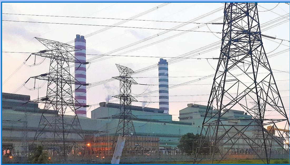
Kapar Power Station
