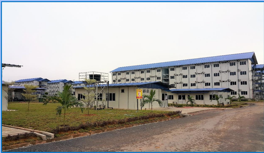
Petronas RAPID Project, Pengerang – Sinopec Camp & TCF
